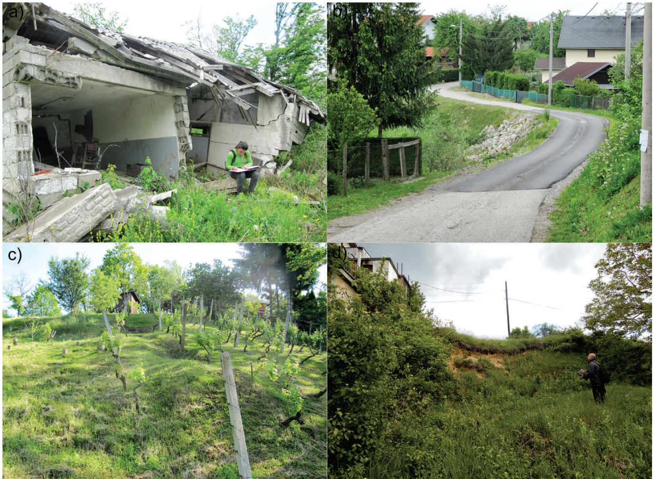
Figure 2. Landslide damage in the Kravarsko area: a) destroyed storage in landslide body; b) road mitigated by rock embankment and “fresh” asphalt; c) damaged vineyard in the main body of a landslide; d) landslide main scarp by a house (photos by HGI-CGS, 2019).
