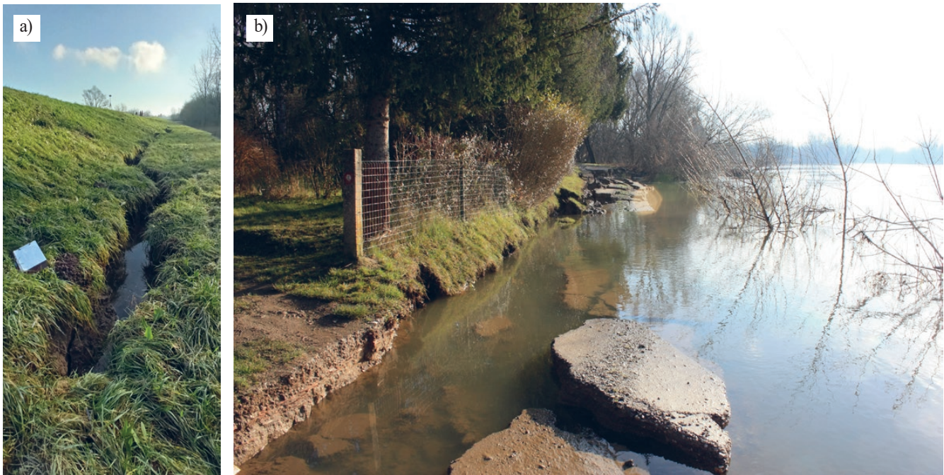
Figure 6. Lateral spreading and associated processes: a) failure of the flood embankment in Sisak (observation point Si-03); b) road failure in Letovanić (observation point RMT-35).
